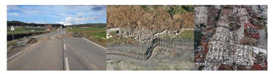
Figure 4. During the 06 February 2023 Pazarcık, Kahramanmaraş, Turkey earthquake, the 3 m offset on the highway and railway and the damage to the buildings can be seen in the region.
